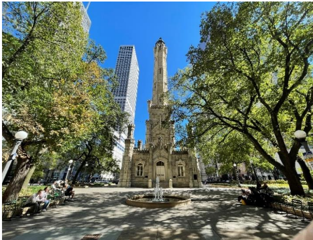
Water Tower and plaza, looking west.
